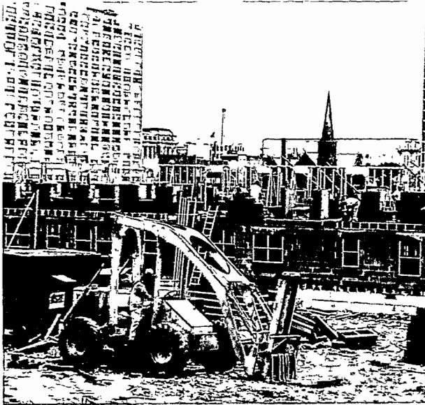
Heavy equipment and construction workers converge on site in Newark, N.J., a cooperative apartment complex, the first housing financed by the life insurance companies billion dollar investment program.
